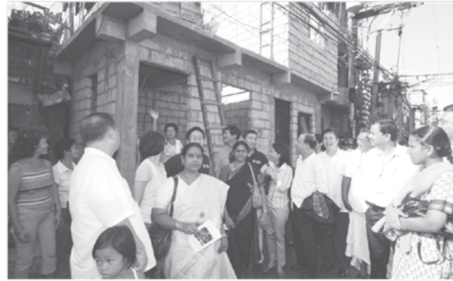
An Indian Rotary Club delegation is shown the construction of homes their club co-sponsored with RCMW
